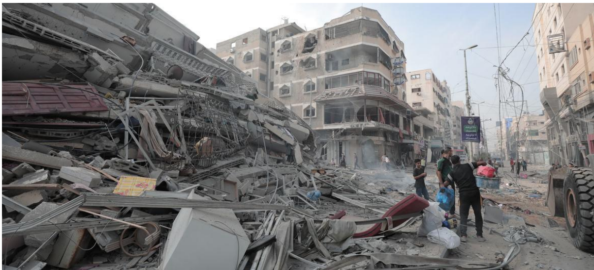
© UNRWA/Mohammed Hinnawi. A building collapsed into the street in Gaza.
