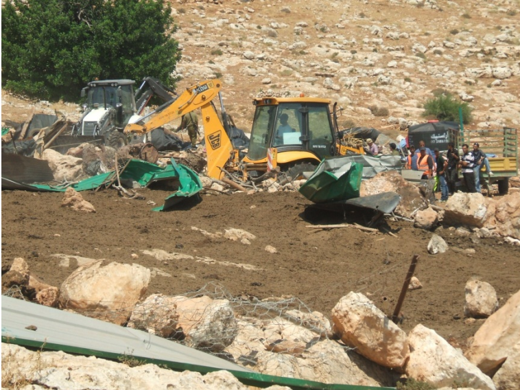
Israeli army demolishing homes in Khirbet Yarza, Jordan Valley, 21 July. Photo: Patricia Mercer, EAPPI.
